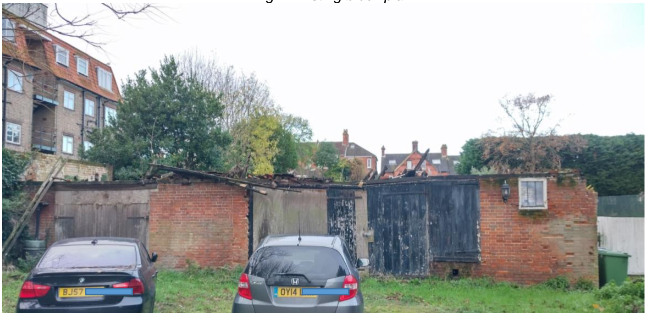
Fig2. Photograph of existing outbuilding
