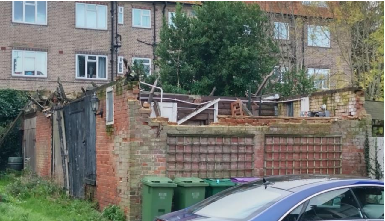
Fig3. Photograph of existing outbuilding
